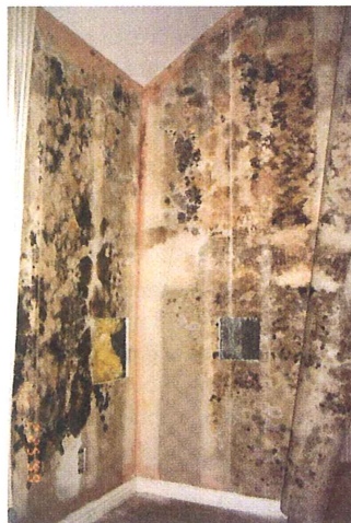
3.5 Figure 3.5: Martin County Courthouse, Stuart, Florida. The HVAC design produced high rates of outside air ventilation but poor temperature and humidity control which contributed to mold and moisture problems, resulting in over $10 million in renovation costs for a three-year-old building.
